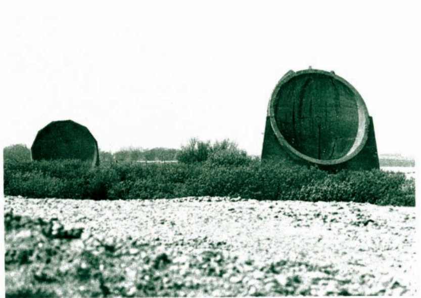
● Fig. 1: Spherical sound 'mirror' listening detectors in Kent (See text).
